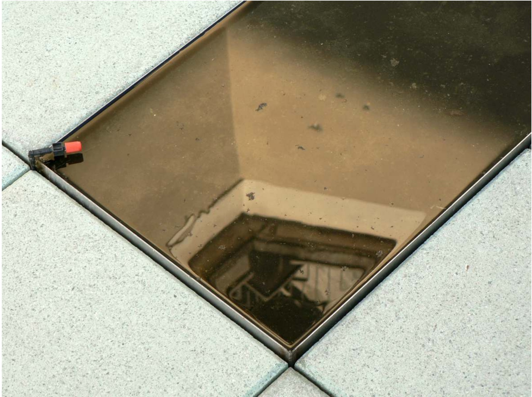
Stainless steel basin containing water, automatic micro-irrigation system.
